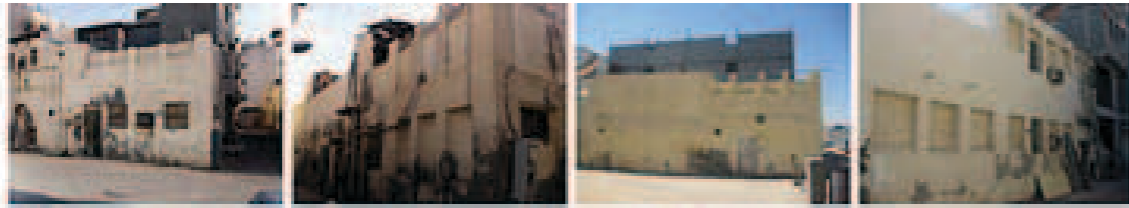
SOME OF THE BUILDINGS TRADITIONAL IN DAWASIR DISTRICT.
